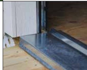
Trac-Rite's zinc-coated sill plate provides protection against sill damage and water intrusion.
